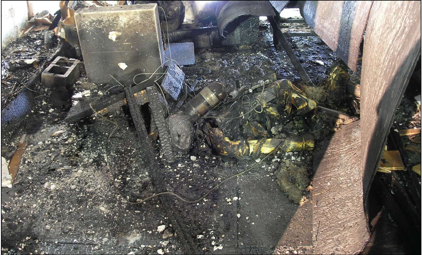
Figure 15: Test 4, first unsprinklered test, damage
