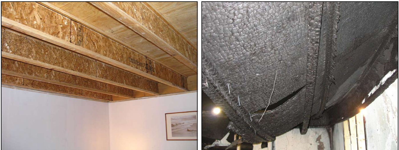
Figure 1: Composite wood joists before (left) and after fire exposure
