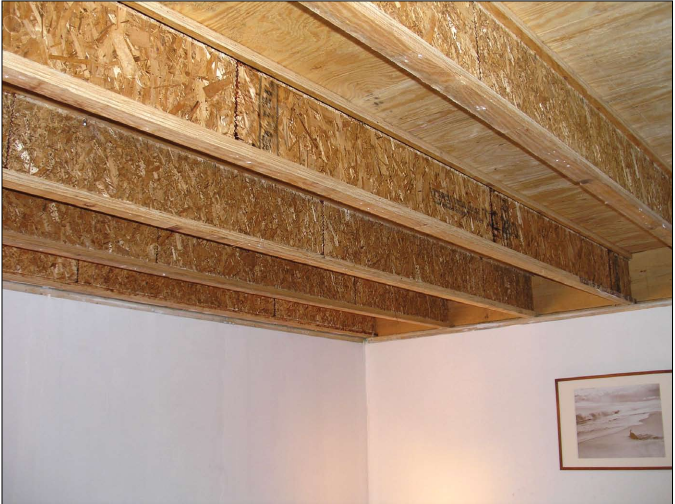
Figure 5: Exposed composite wood joists representing main level floor assembly
