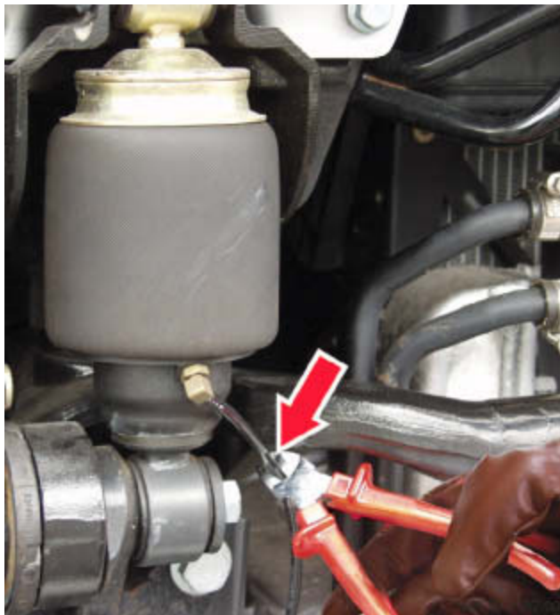
Cutting air line at air bellows
