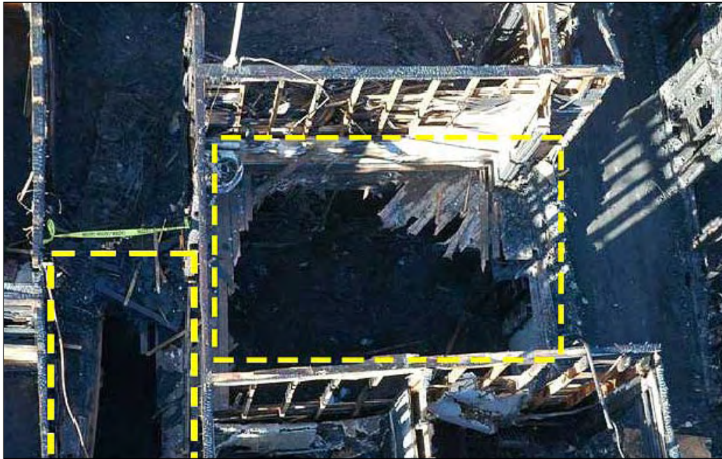
Figure 9. Overhead Photo of Collapsed Areas of Third Floor.
