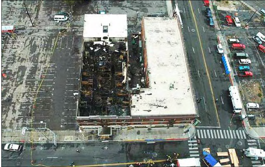
Figure 14. Extent of Fire Damage—North Wing.
