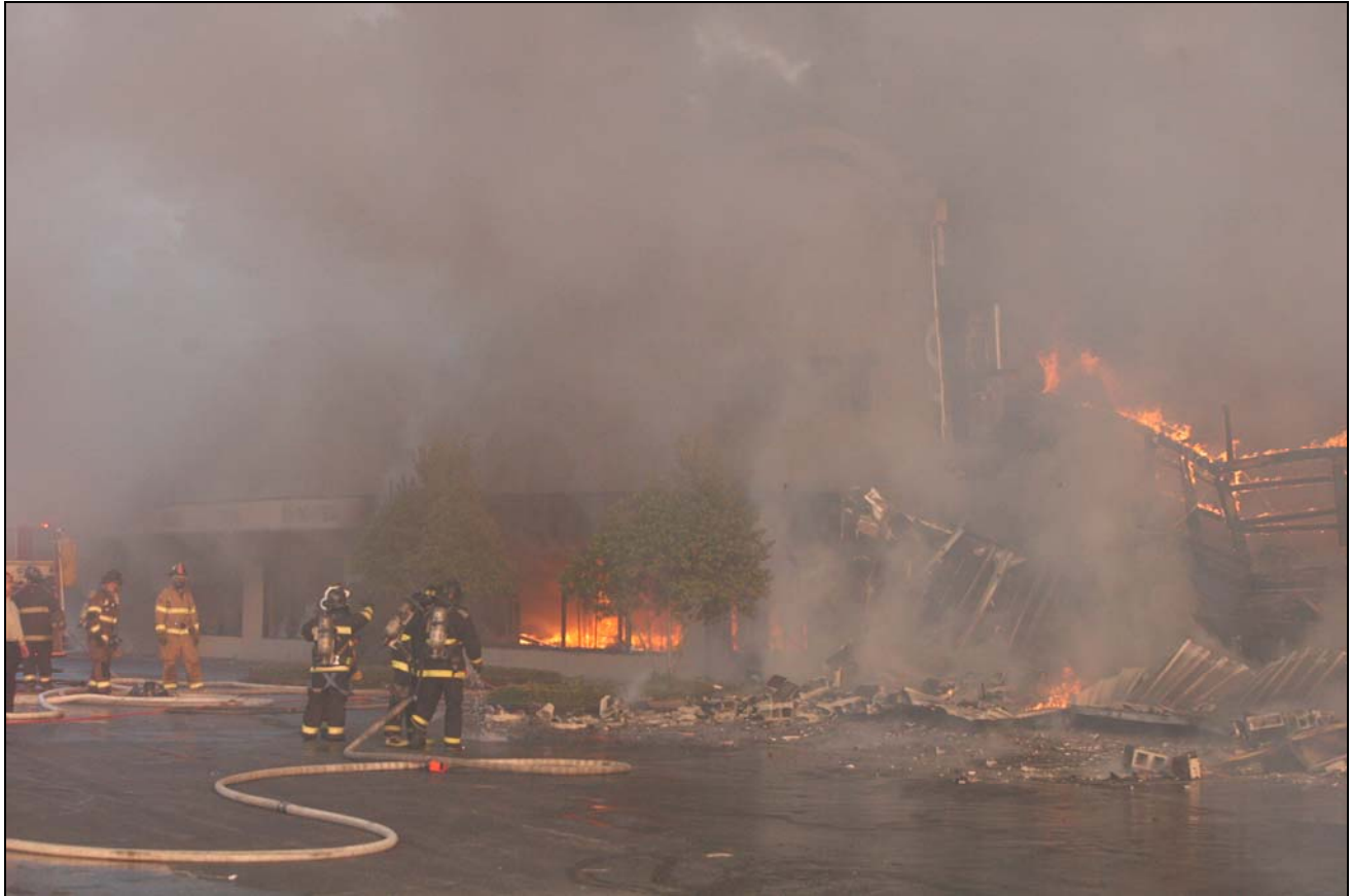
Photo A-4: Time approximately 1951 hours. Front façade beginning to collapse. (Photo courtesy of the Charleston Post and Courier.)
