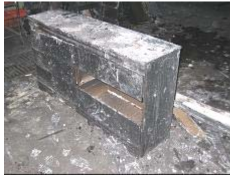
Dresser (post fire)
