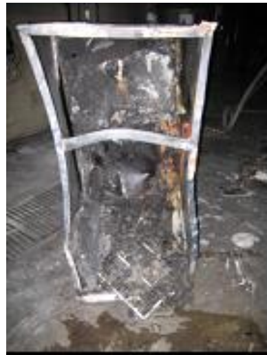
Refrigerator (post fire)
